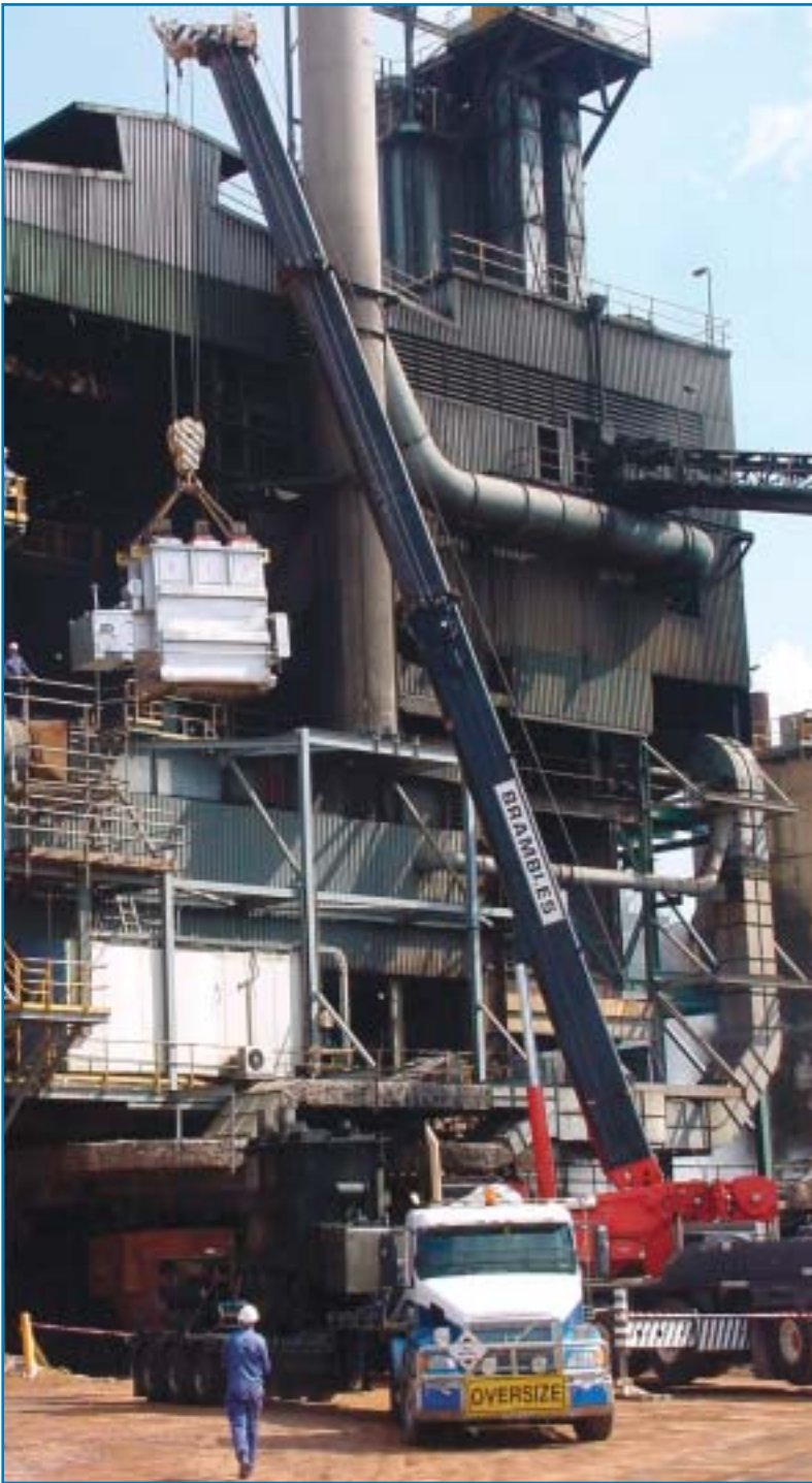
An intricate emergency remove and replace job.
