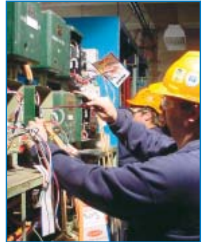
Repairs to control systems.
