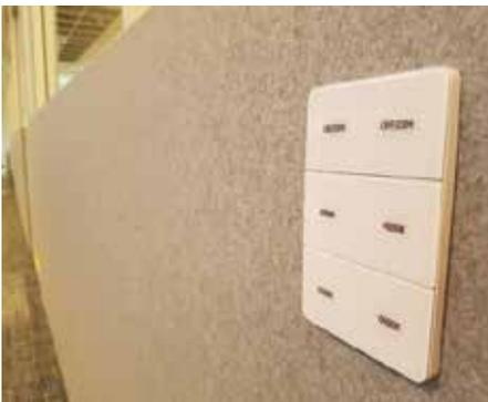
The PSB facility was also a 100% LED lighting project which required different type of DALI lighting control system to enable it to fully connect back to a central location through the DPTI network which allows for monitoring and reporting of all light fittings for maximum efficiency and user safety.
