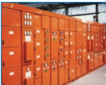
Typical arcfault design.
