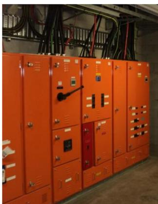
In April 2012, a TEGG report completed by Nilsen at **Westfield Strathpine** identified that PFC units in two main switchboards were not operating to maximum effect. Nilsen arranged immediate replacement of the PFC unit components, ensuring optimum PFC of the switchboards.
