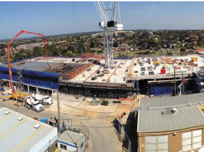
New Telstra datacentre during construction.
