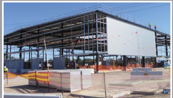
Defence Logistics Transformation Project at Moorebank
