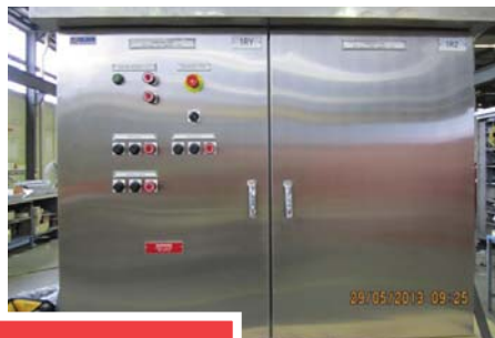
Stainless steel outdoor switchboards.
