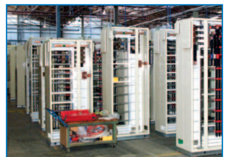
Being fitted out
