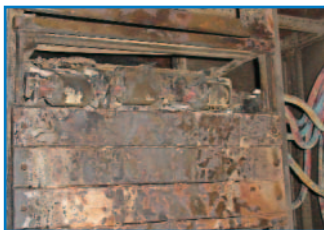
A tough repair job
