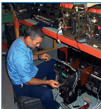
Circuit Breaker Rebuilds
