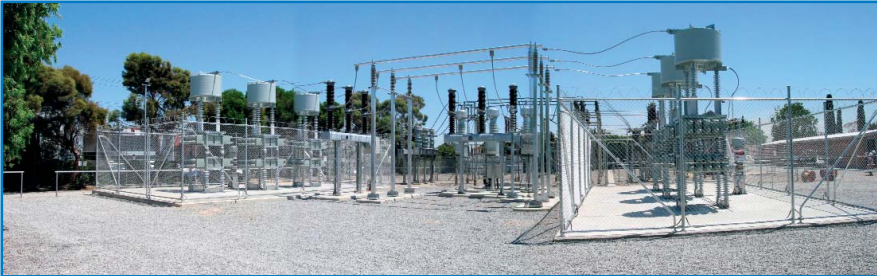
HV Reactor Installation
