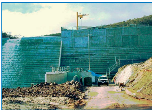
Water Catchment Electrics
