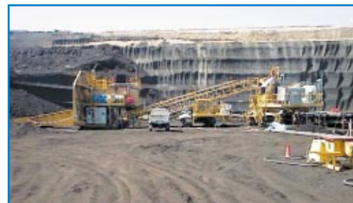
Crusher Installation, Morwell Vic
