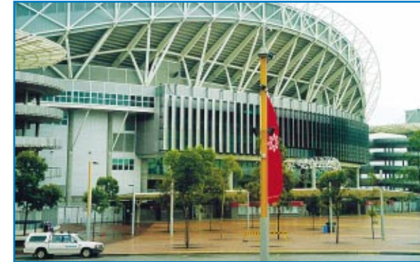
Stadium Australia Refurbishment
