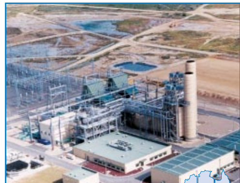
Pelican Point Power Station
