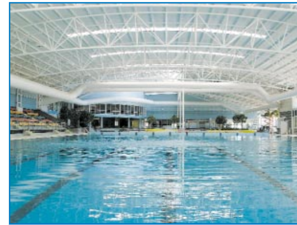
Bunbury Aquatic Centre Electrical Installation
