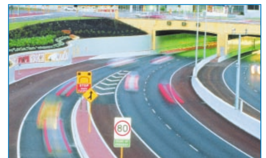
Graham Farmer Freeway lighting, photo courtesy of WA Dept of Main Roads
