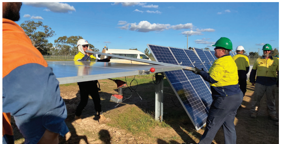
Last Panel being put in place at Darlington Point
