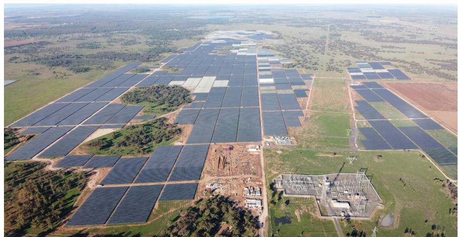
Darlington Point Drone East Facing
